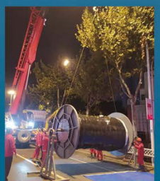
某市DN500热力管道柔性内衬修复
